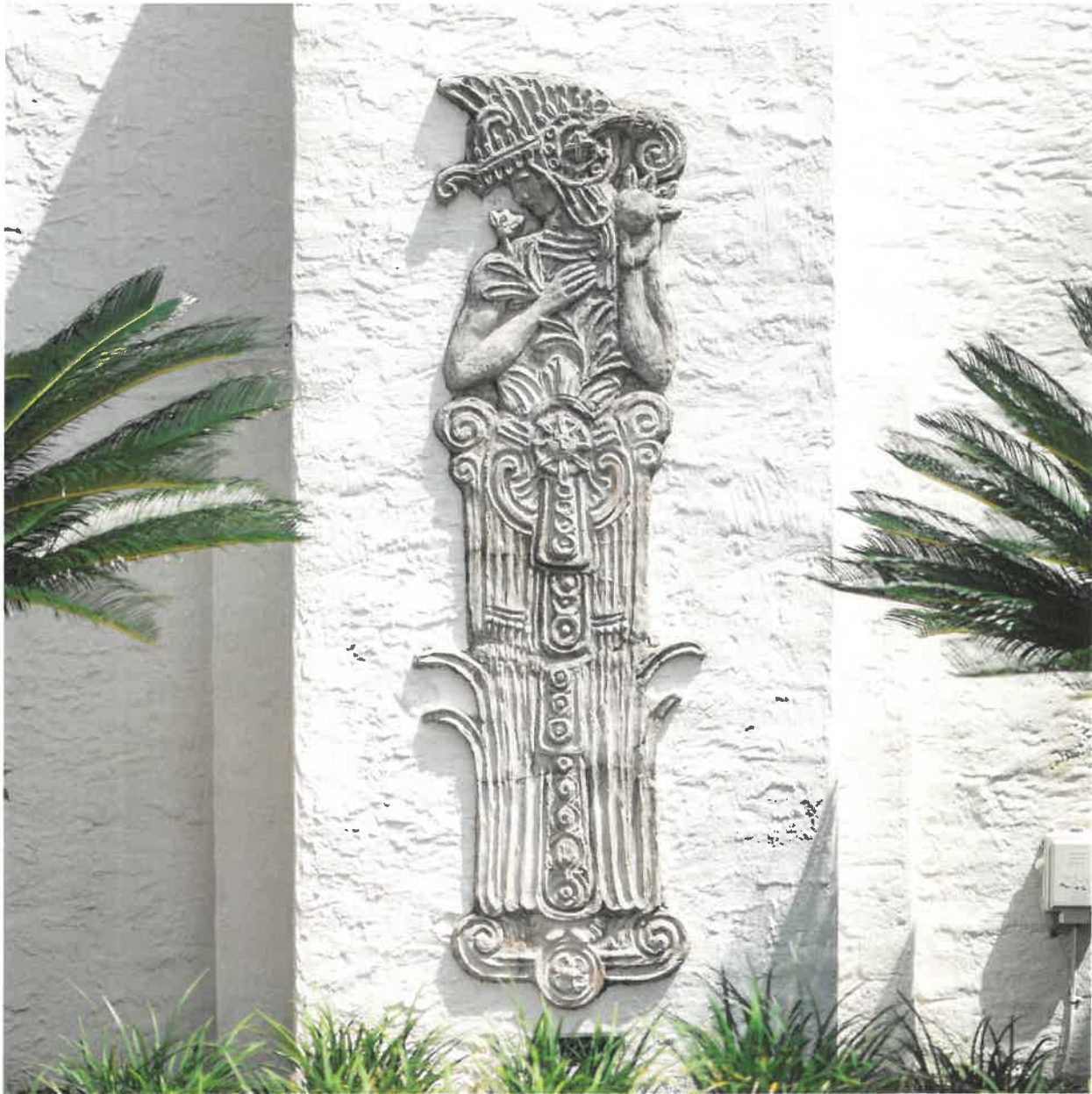
Both images show concrete reliefs, which are decorative designs Jules Andre' Smith made by carving into specially prepared surfaces. Over 2500 concrete reliefs appear on walls, doorways and pathways of the Art & History Museums of Maitland.
